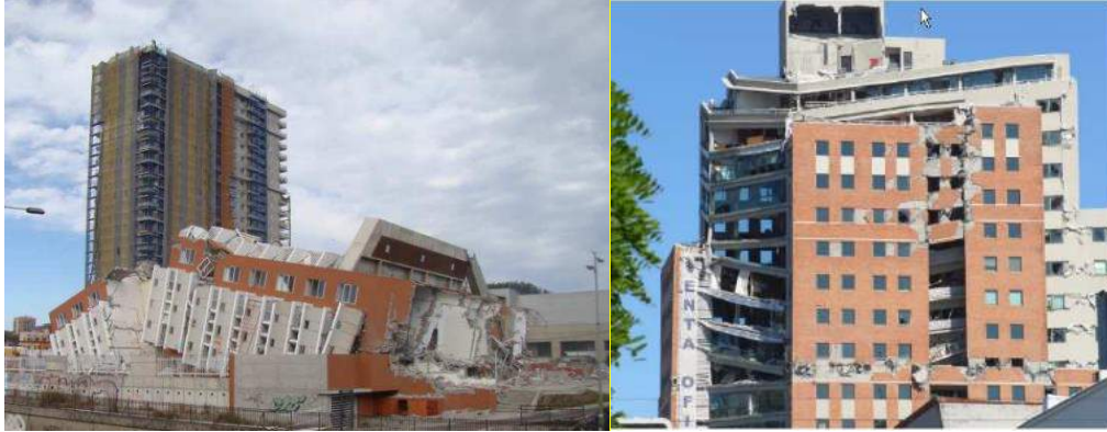
Figure 5 – Alto Rio Tower (fully collapsed, left) and O Higgins Tower (partially collapsed, right) [2]
