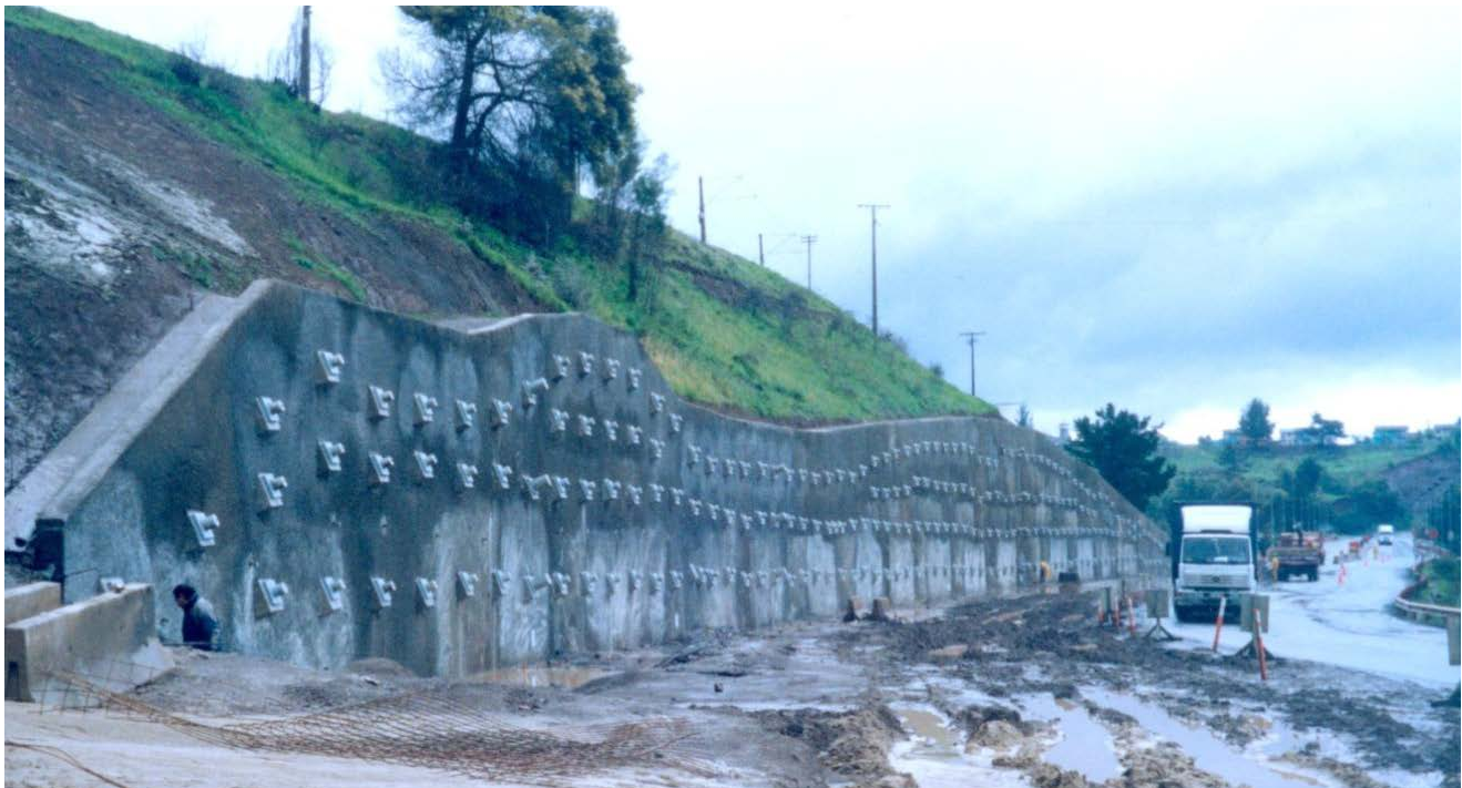
Fig. 5 – Anchored Wall building just finished.
