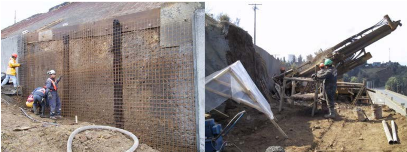
Fig. 3 – Excavation, draining strips, mesh and shotcrete. Execution of ground anchors.
